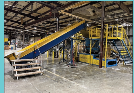
60" Diameter Densifier, 288 KW Motor
