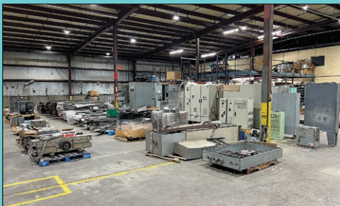
Large Quantity of Square D Transformers & Breaker Panels
